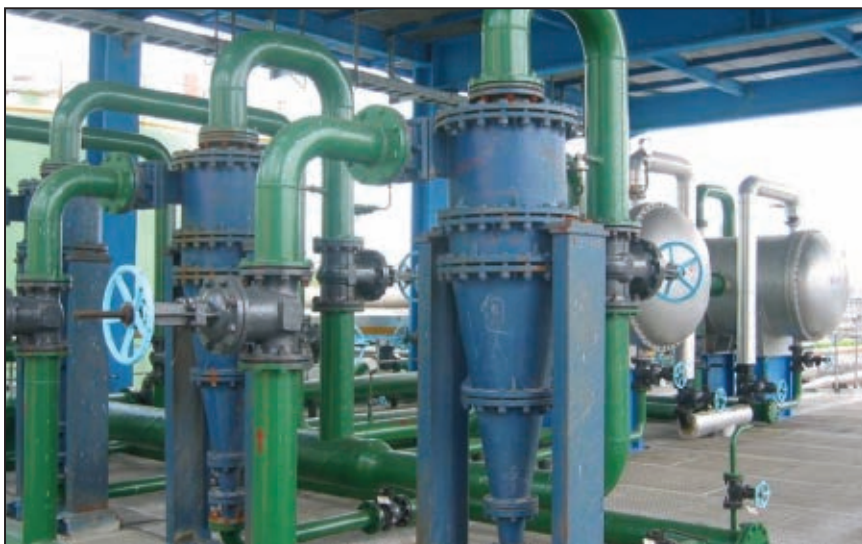
FIGURE 4. A de-oiling hydrocyclone is shown with an air cooler in a plant facility
