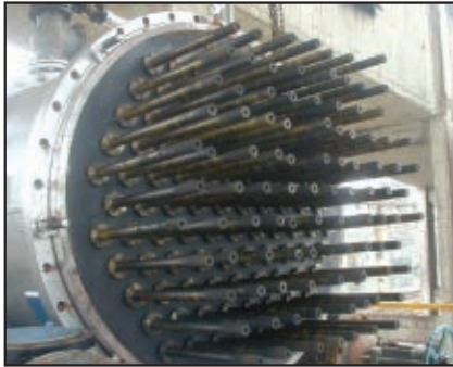
FIGURE 6. A de-oiling hydrocyclone helps improve coke-cooling efficiency
